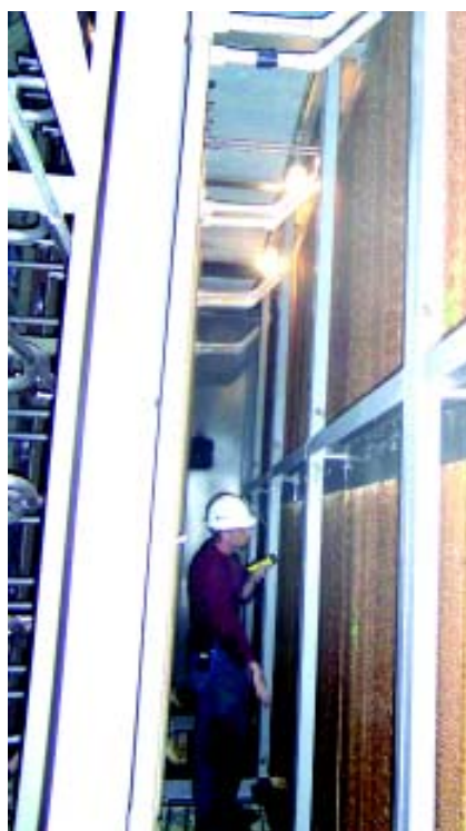
ABOVE: Evap inspector checks for gaps in the media and signs of deterioration.
