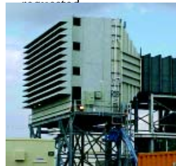
RIGHT: Evaporative cooler section is typically located behind filter section.
